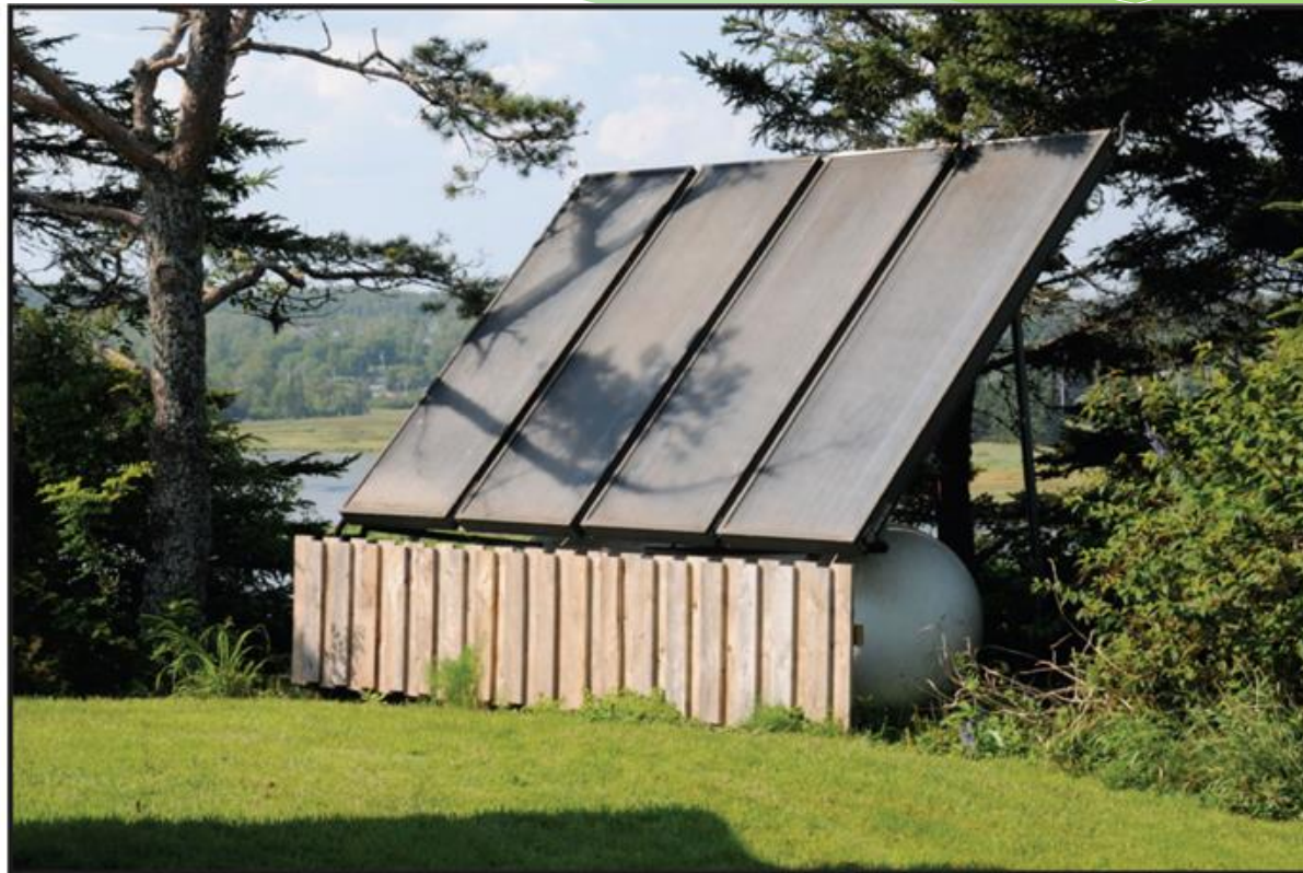
Figure 8.5: Flat plate solar collector installation.
